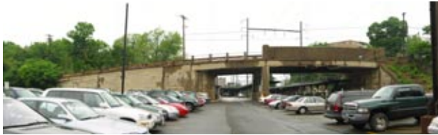
Existing Greenwood Avenue Bridge
