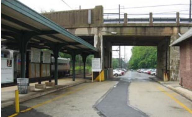
On-Site Road Under Greenwood Avenue Bridge
