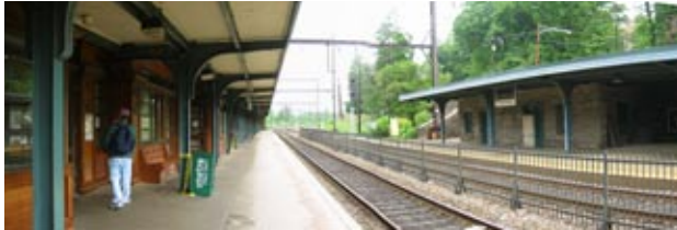
Existing Station Platforms
